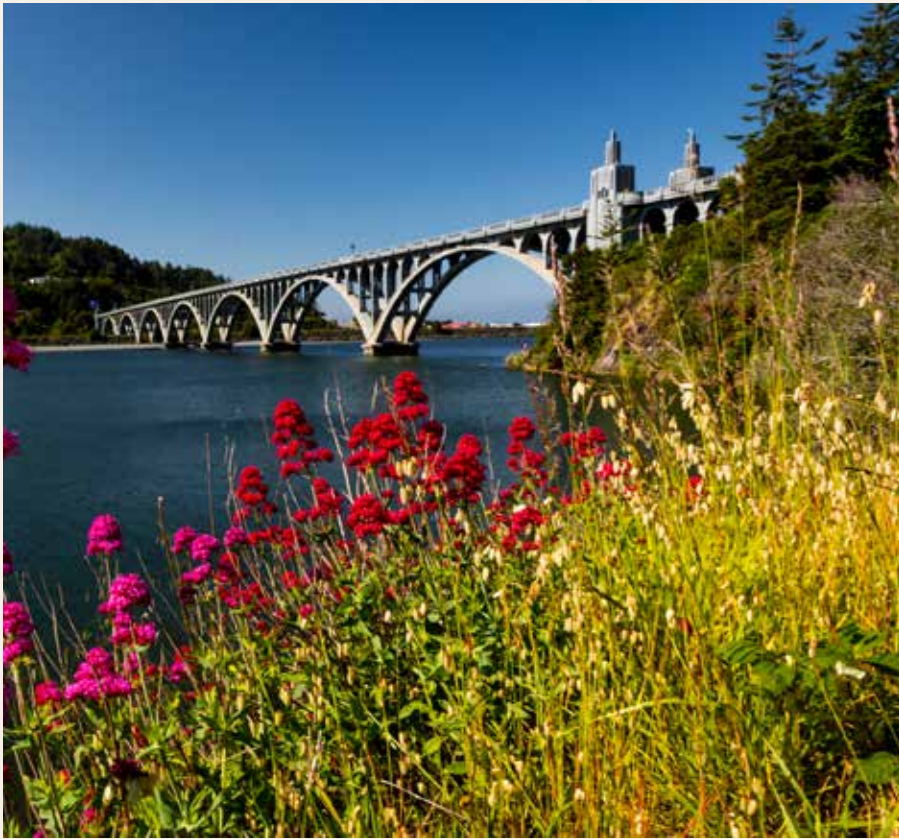
L.L. Patterson Memorial Bridge.
